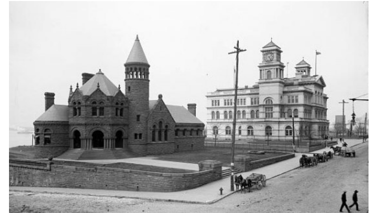
Image of Original Cossitt Library (left/foreground) in 1910 from Historic-Memphis website
